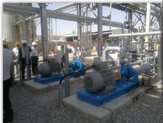
Darquain Early Production Unit, 50,000 BBL/day Light Crude Oil Booster Pumps
