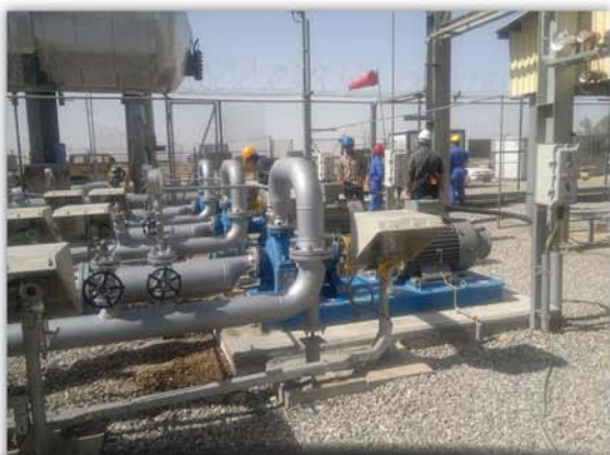
Darquain Early Production Unit, 50,000 BBL/day Light Crude Oil Booster Pumps
