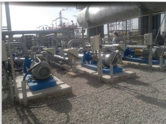
Darquain Early Production Unit, 50,000 BBL/day Light Crude Oil Booster Pumps
